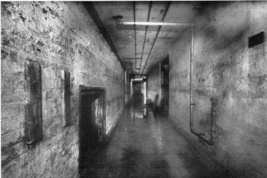
The main spine corridor on the lower level after removal of an inch of slime. Photo John Smiles
